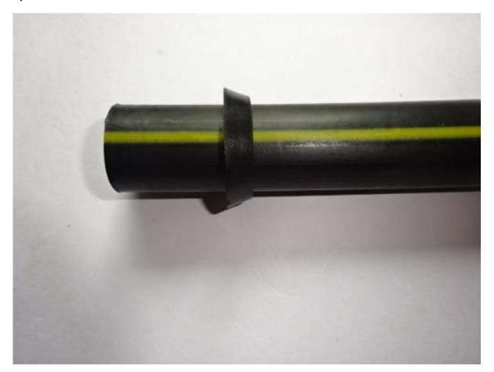
Fit the 25mm grab ring over the 'diverter' sub-duct.
