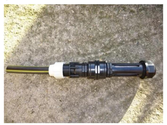
At the end of the section of the diverter sub-duct fit the SDMB5 Guard 1.
