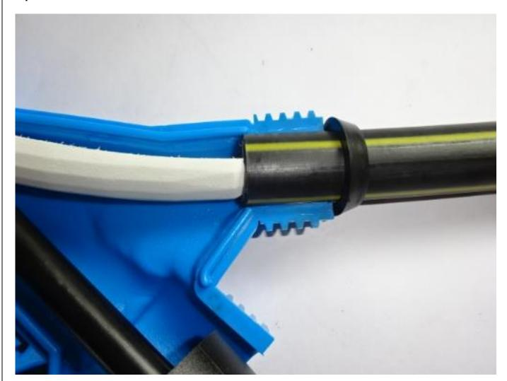
Position the 'diverter' sub-duct into the diverter body.
