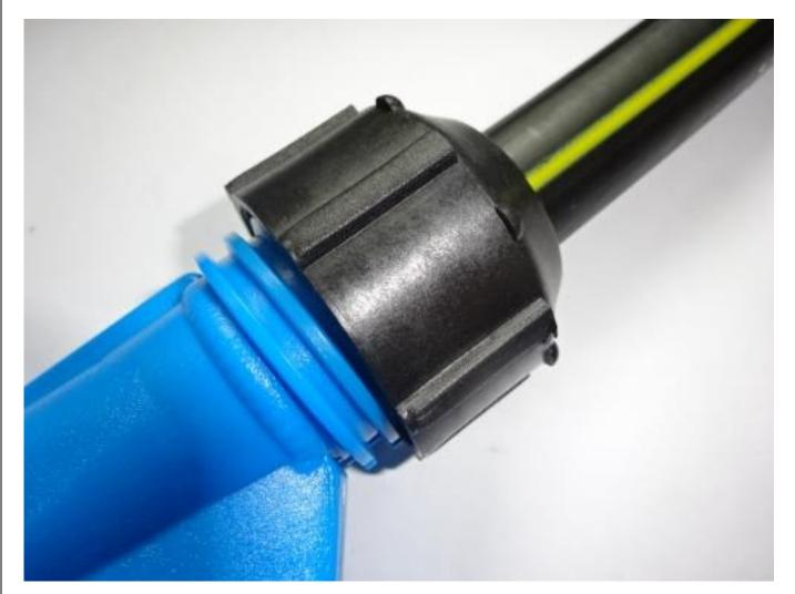
Tighten the lock nut on the diverter sub-duct.
