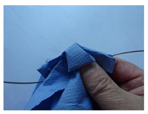
Remove the grease from around the optical fibres.
