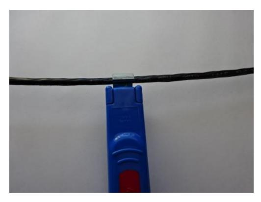
At a point 150mm from the end of the cable apply a circumferential cut to the cable.
