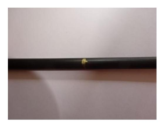
Determine the amount of sheath to be removed and at the required distance mark the cable sheath.
