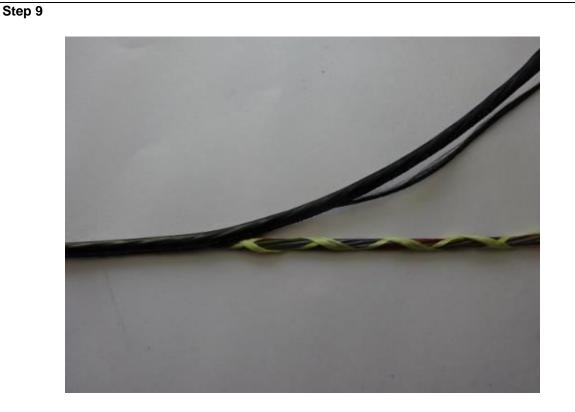
Remove the cable core from the sheath.
