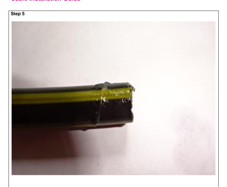
Smear some silicone grease around the bottom of the 14/10mm mini-duct.
