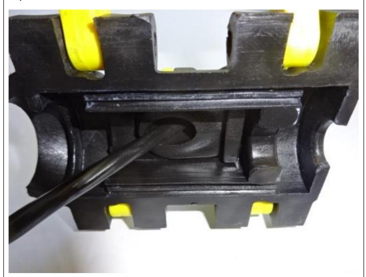
Feed the overblown cable through the top half of the closure body and through to the end of the 14/10mm mini-duct.
