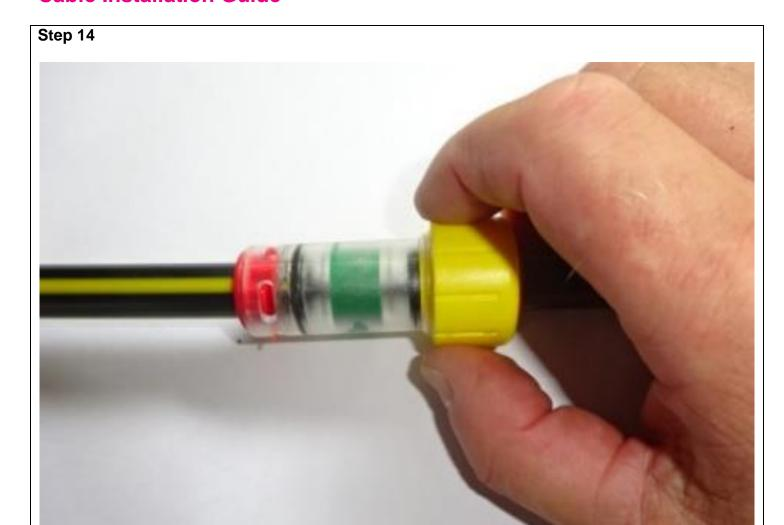
Activate the Water block by tightening the yellow nut.
