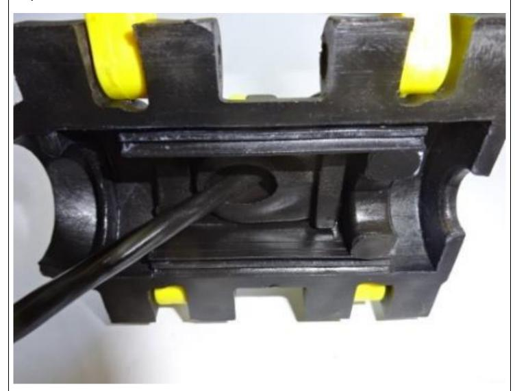
Feed the overblown cable through the closure body, 14/10mm mini-duct and second closure body
