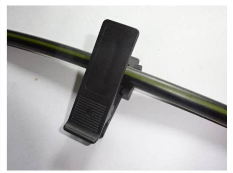
At a point 300mm from the Swept T Closure cut the 14/10mm mini-duct.
