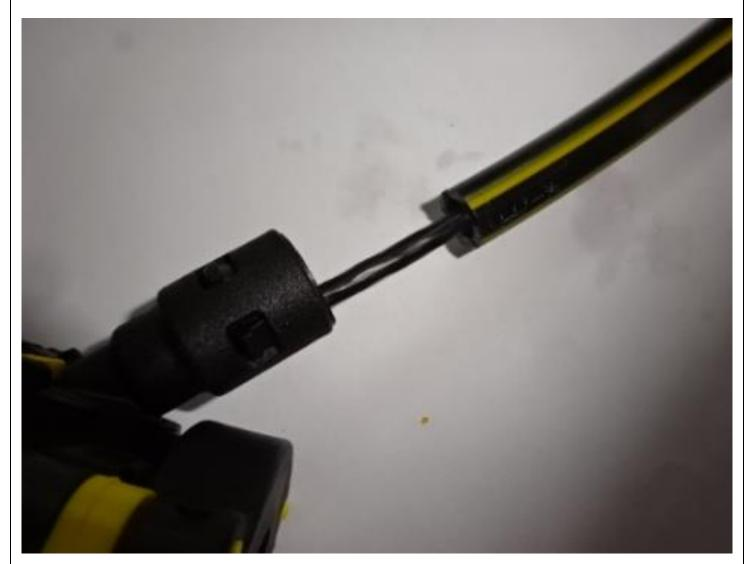
Remove the tool from the 14/10mm mini-duct.
