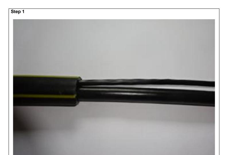
Ensure sufficient overblown cable has been blown out of the sub-duct to reach the final destination.
