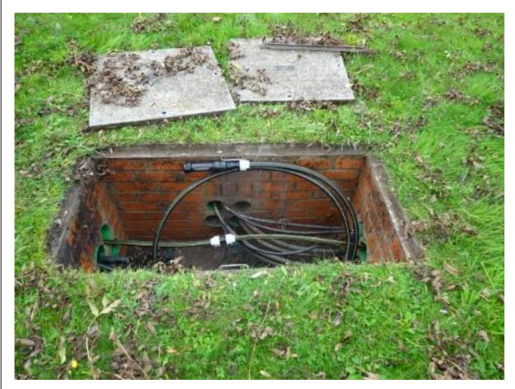
Position the SDMB5 Guard 1 in the manhole.
