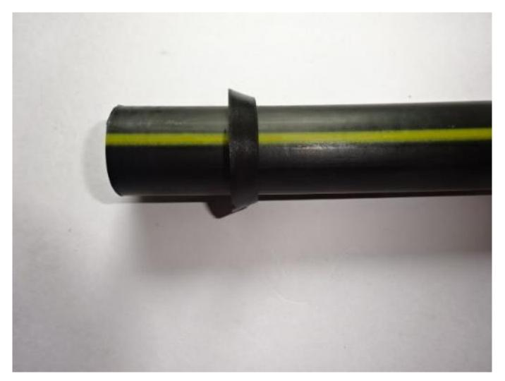
Fit the 25mm grab ring over the sub-duct.
