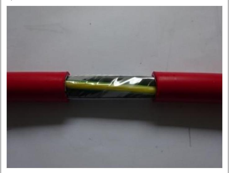
Remove the 150mm section of cable sheath
