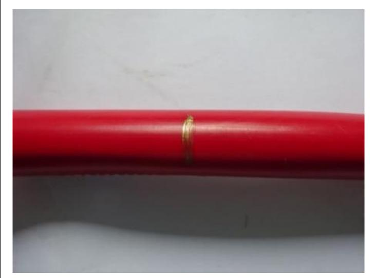
Determine the amount of sheath to be removed and at the required distance mark the cable sheath.
