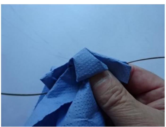
Using a cloth with a suitable cleaning fluid e.g. IPA remove the grease from around the optical fibres.
