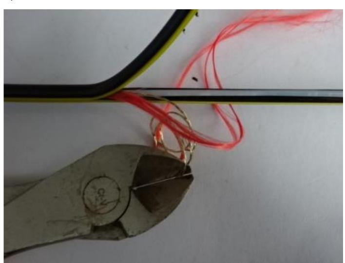
Cut the steel wire strength member to the required length.
