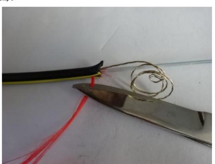
Using scissors cut the water swellable yarn(s) off. Using scissors cut the water swellable yarn(s) off.
