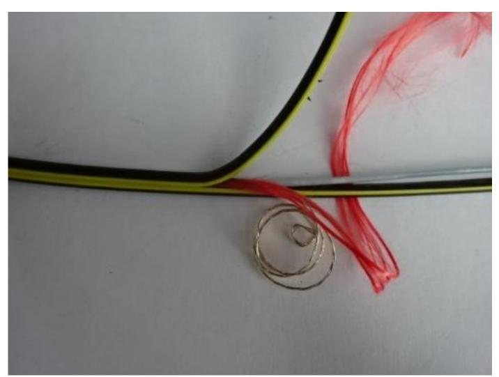
In the event that cable anchoring is required within the optical fibre joint remove one of the steel wire strength members from the split sheath using two pairs of pliers. If not then go to step 8.
