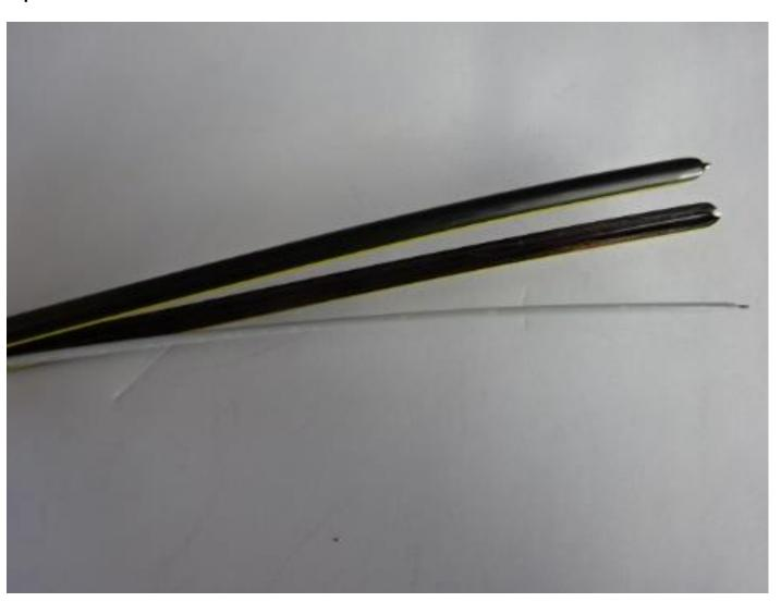
Split the two halves of sheath to expose the fibre tube.
