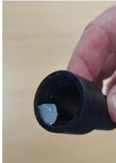
Grease the seal body that has already been installed on the end of the 16mm sub duct, ready for the fibre seal to be installed into it. This should be rubbed around the inside of the recess in the seal.
