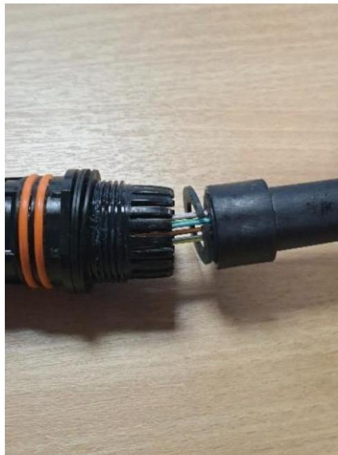
Thread the fibres through the gland body and insert the seal making sure not to trap any fibres inside the gland body.
