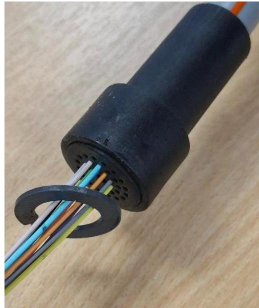
Now push the fibre seal into the seal body already installed onto the sub duct. Ensure the top of the seals are flush. Once this has been completed. Install the split washer on top of this seal.
