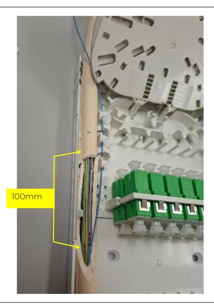
Identify the previously prepared entry point for the feed cable. Then Install and fix the cable to the PBI-16SC. And tighten cable ties to secure cable.
