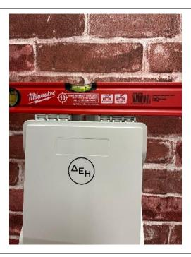
Mount the products using the screws & ensure both products are level.
