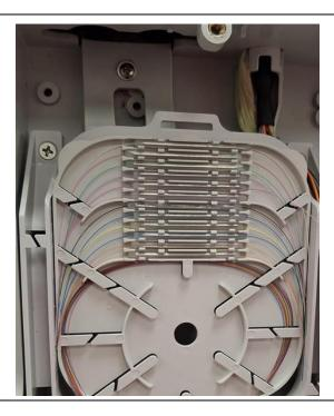
Splice the incoming cable to the existing pigtails, using your company's preferred method. Place the splices in the tray positions as shown.
