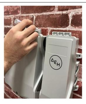
Mark on the wall using a marker, the locations of the mounting positions.
