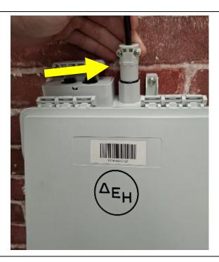
Secure the 2 plates back together and clip the gland back into the BEP.
