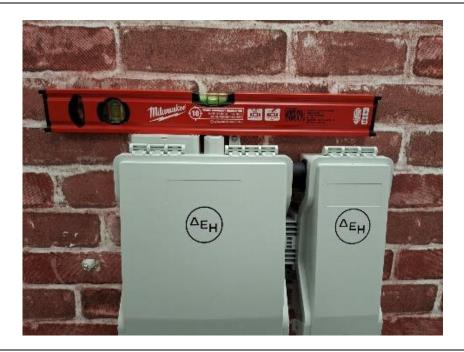
Mount the products using the screws and ensure both products are level.
