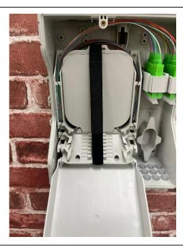
Place the splice tray cover back on to the tray, wrap the velcro around and lock the splice area up.
