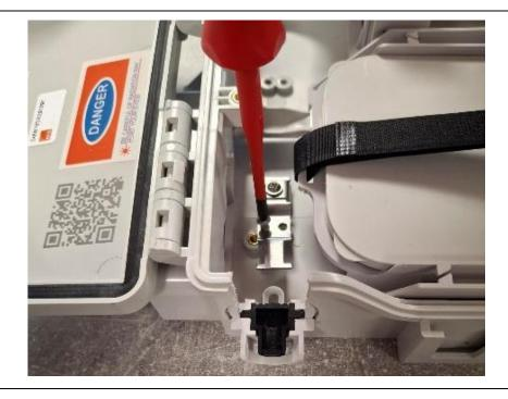
Secure the cable restraint bracket using the screws supplied in the kit.
