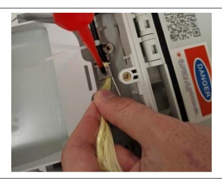
After bringing the cable through the inline seal, anchor it in place by using a cable tie. Use the kevlar from the cable and wrap it around the anchor bracket 3 times.
