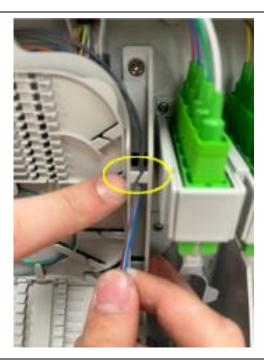
Bring the incoming cable elements into the routing area, ensure that the elements are stripped after the point highlighted.
