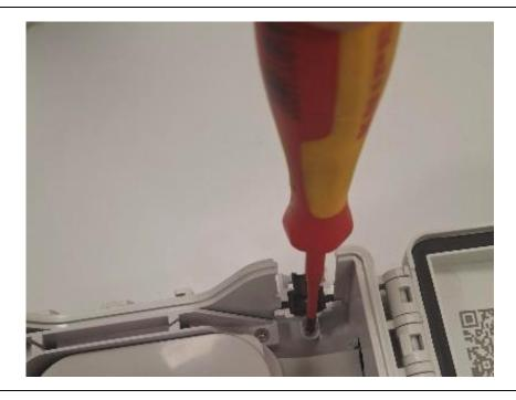
Secure the bottom half of the inline cable seal to the BEP, using the screw provided in the kit.
