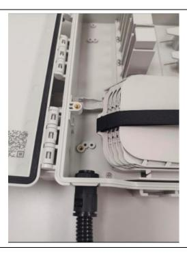
Place the gland into the BEP and attach the nut on the back of the corrugated tube.
