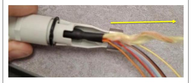
After sliding the gland back over the cable, measure out 50mm of Kevlar to use when coiling the cable.
