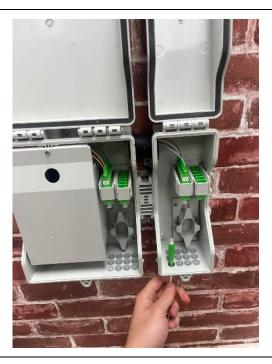
Push through the rubber grommet through. Then bring in the drop cable.
