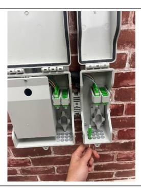
Push through the rubber grommet through. Then bring through the drop cable.
