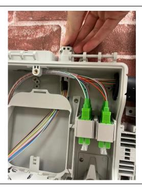
After clicking the gland back into position, route the elements down behind the trays.
