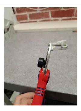
Cut the rubber grommet open, this will depend on the cable diameter.
