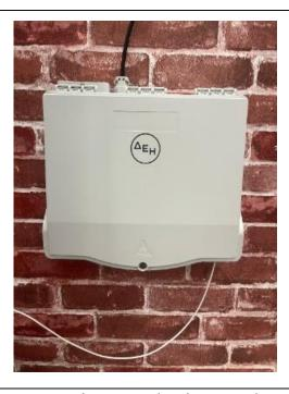
Close the lid of the BEP and screw it shut ,using the key.
