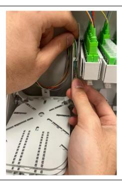
Route the fibres up onto the trays, make sure that the elements are stripped at the point shown.
