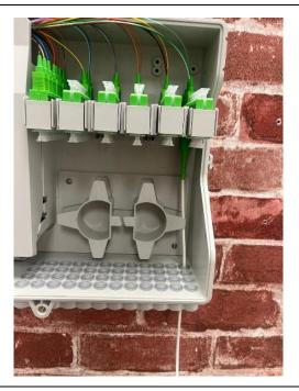
Connect the drop cable into the patch panel and plug it in. It should look like this.
