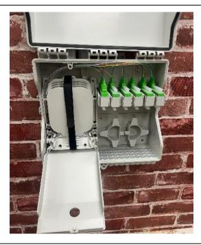
Place the splice tray cover back on to the tray, wrap the velcro around and lock the splice area up.
