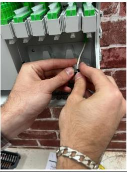
Place the rubber grommet over the drop cable and place the plastic housing over the grommet. Click into place.
