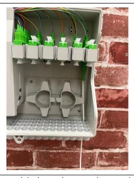
Connect the drop cable into the patch panel and plug it in. It should look like this.
