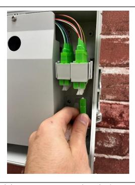
Then feed the rubber grommet back into the BEP going to opposite way as before. Click the drop cable in the required position.
