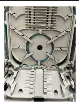
Splice the incoming cable to the existing pigtails, using your company's preferred method. Place the splice holder in the position as shown.
