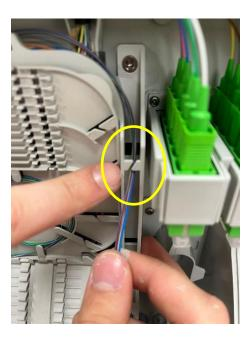
Bring the incoming cable elements on to the tray, ensure that they are stripped at the position pointed out.
