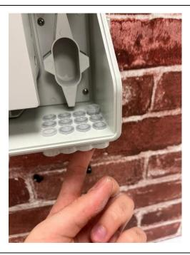
Push through the rubber grommet as shown. Then unclip the rubber from the plastic housing & open the plastic.
