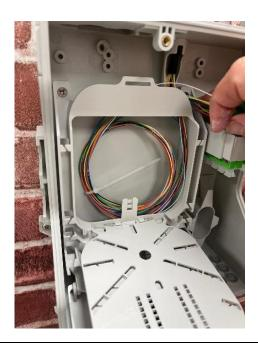
Coil the elements as shown, going clockwise.
