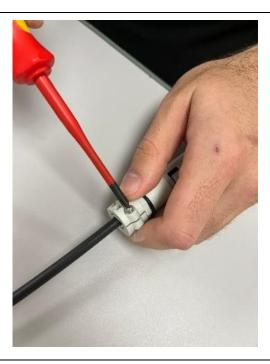
Fully tighten the two gland plates together.
