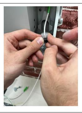
Place the rubber grommet and plastic housing around the drop cable. Click it shut, then feed it into the BEP.
