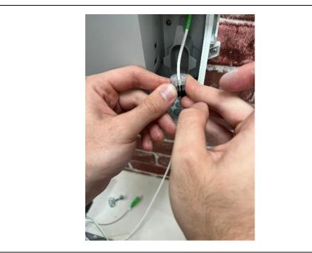
Place the rubber grommet and plastic housing around the drop cable. Click it shut, then feed it into the BEP.
