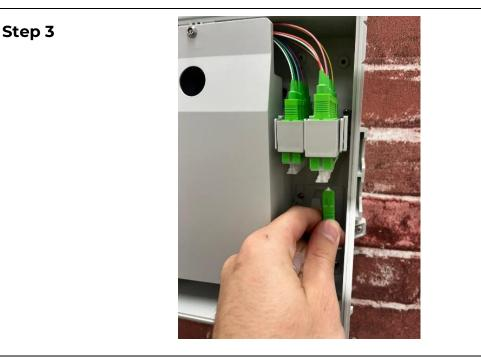
Then feed the rubber grommet back into the BEP going to opposite way as before. Click the drop cable in the required position.
