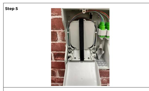
Place the splice tray cover back on to the tray, wrap the velcro around and lock the splice area up.
