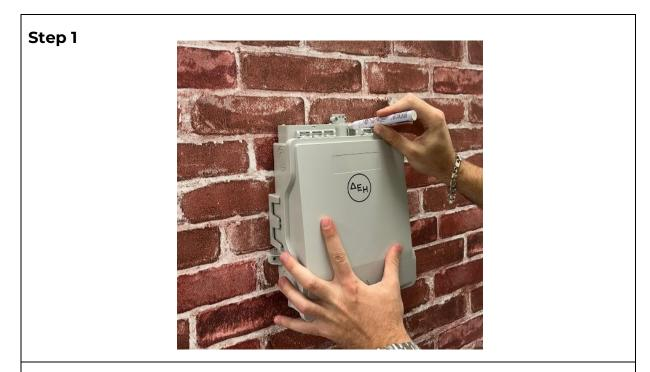
Mark on the wall using a marker, the locations of the mounting positions.
