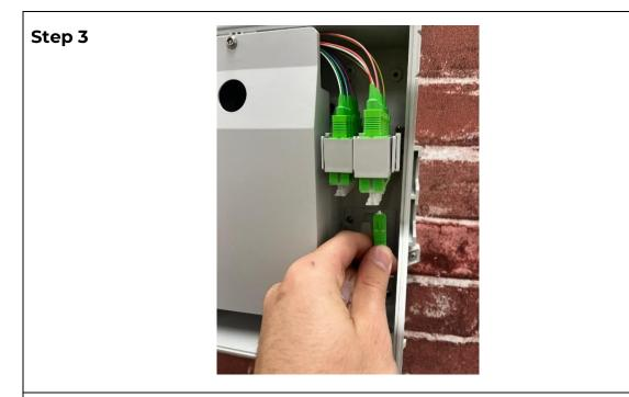
Then feed the rubber grommet back into the BEP going to opposite way as before. Click the drop cable in the required position.
