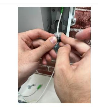
Place the rubber grommet and plastic housing around the drop cable. Click it shut, then feed it into the BEP.
