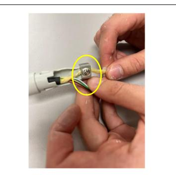
Feed your cable through the gland, anchor the aramid under the screw. Ensure that there is space under the metal and the screw is not fully tightened before trying to slot the aramid underneath it.
