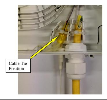
• Secure cable with Cable Tie hand tight only in position shown. Cut off Cable Tie tail using Flush Cutting Tool.
