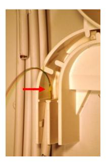
Remove the protective sheath from the BFU to a point 25mm from BFT butt.
