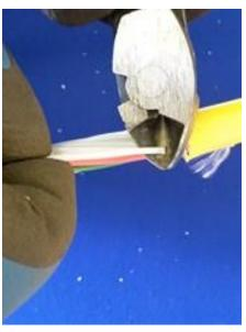
Identify the element containing the fibres to be spliced and cut it close to the output side sheath butt.
