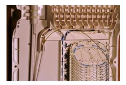
• Install 4 Fibre BFU into the nominated tube and allow an additional 2,5m of BFU for fibre management within the closure.
