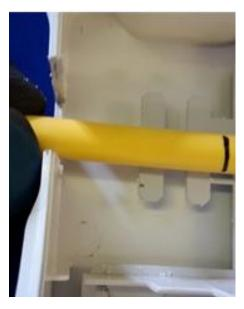
• Place the input side of the cable into the bottom port slot and mark the sheath just above the cable retention bracket.
