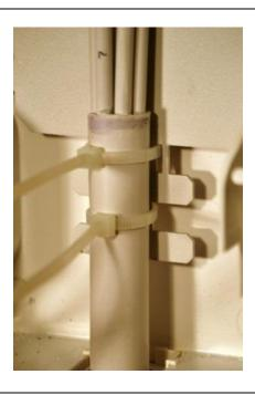
• Retain to the retention lugs in the base of the closure using the large cable ties supplied.
