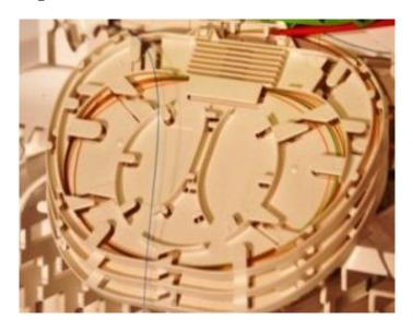
• Manage the spare fibres into the central storage area via the outside fibre track.
