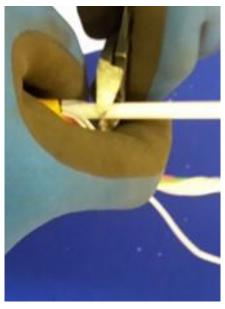
• Cut the strength member close to both sheath butts and remove. Also remove any dummy fillers and rip cords.
