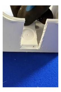
• Snap-off remaining material to form a cable access slot.
