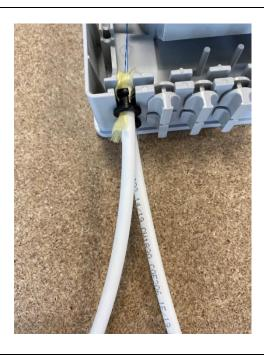
• Alternatively, you can place two cables into the Individual cable breakout.
