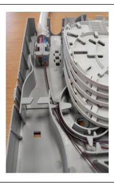
• Following the same steps as Fibre routing – Upper universal breakout Internal tubing, pages 30-35. Ensure there is 1.5m of fibre from the tube butt.
