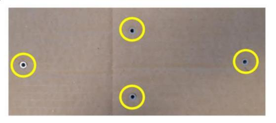
Drill 4 holes as marked using the 5mm drill bit and fit wall plugs into the holes.
