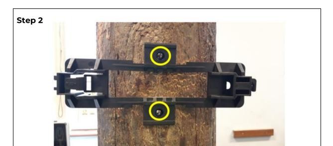
• Screw bracket to pole using screws provided.
