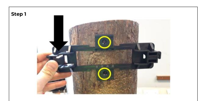
Place the bracket against the pole in the final position as required and mark 2-hole positions as shown.
