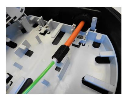
• Put about one and half turns of foam tape at the end of the out sheath.
