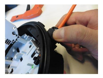
• Tighten the sealing nut of the gland.
