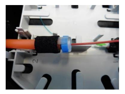
• Wrap about one and half turns of foam tape around the Miniduct Seal.
