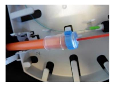
• Mount the Miniduct Seal onto the mini duct following the installation instruction.
