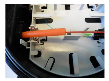
• Carefully put the fibre element and mini duct into the closure through the gland.
