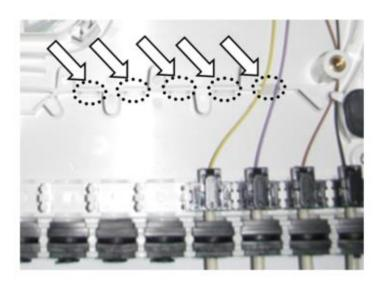
• ... just breaking the highlighted breakable walls.
