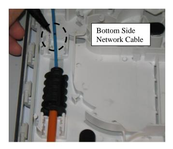
• Mark the cable on the top side of the circled cable clip saddle.
