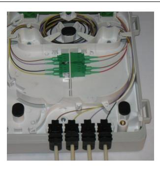
Or to park the modules (without the external sheath) of preconnectorized Customer Cables.
