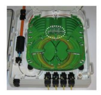
• Alternatively, a bare fiber splitter can be installed in the bottom or the top tray.
