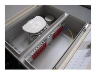
• Route the patch cord through the cable gland at the bottom.
