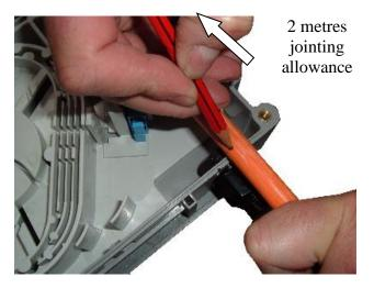
• At the outside wall, mark a butt position on the input cable level with the top of the cable gland. Allow a further 2 metres for the jointing allowance for conventional cables and a further 200mm for a Blown Fibre cable.
