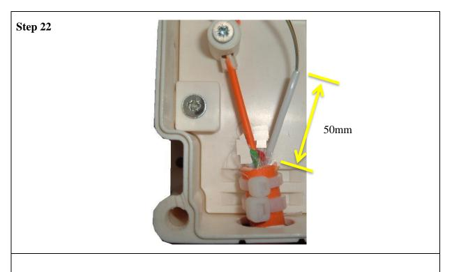
• Strip the cable element to expose the fibres approximately 50mm from the cable butt.
