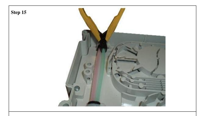
• If the cable is in line, cut the required tube as close to the second cable butt position as possible.
