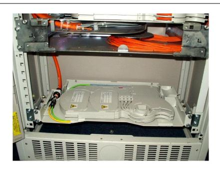
• Using 4, M6 x 12mm screws (3) and 4, Nylon Washers (5) fit shelf and cable in position.
