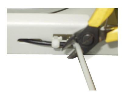
• Secure the CSM to the sidewall using the 2 cable ties (6). Remove excess length of cable ties using a 'flush cutter'.
