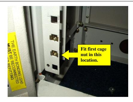
• Select the rack mounting position for the shelf and fit 4 Cage nuts (4) into the rack uprights.
