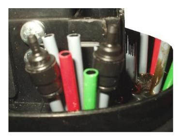
Install Tube Water Blocking Connectors (BT Item Code: 075692) to each of the tubes.
