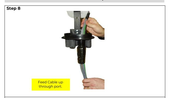
Carefully feed the cable up through the port. Push the cable up until the butt position is accessible.
