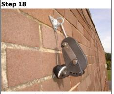
Attach a suitable pulley to the Mounting Clamp.
