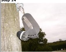
Attach a suitable pulley to the Mounting Clamp.
