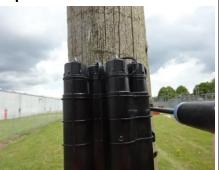
Re-attach the connector housing to the base. The housing is designed for either top or bottom entry of the drop cables.
