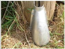
Fit the capping adaptor to the base of the pole.
