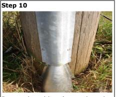
Protect the cable going up the pole with the steel or plastic capping.
