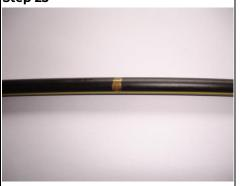
Determine the length of cable required to link the tension clamp to the CBT External Customer Termination Box. Mark the cable at this point and add an extra 3m.
