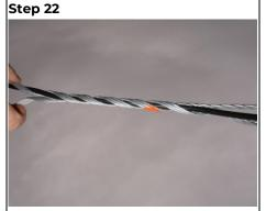
Fit the helical tension clamp to the cable and mounting clamp at the cable dispenser pole.
