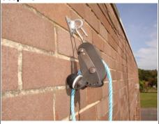
Pass the pulling bond through the pulley at the remote pole/house.
