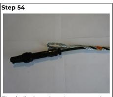
Fit a helical tension clamp around the drop cable. Note the position of the clamp relative to the connector.
