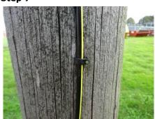
Secure the feeder cable down the pole using pole cleats.
