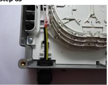
Insert the drop cable through gland and position approximately 65mm from the lowest face of the box.
