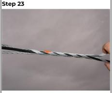
Pull the cable to the required tension and fit the helical tension clamp at the pole/house.
