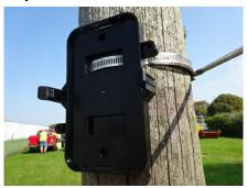
Attach the base to the pole using the steel banding provided. Alternatively, the base can be attached to the pole using wood screws.
