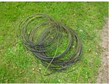
Remove and fleet sufficient cable from the drum to enable the cable to be installed into the u/g joint. Step 6
