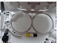
If the wrapping is done correctly there will be no excess tube.
