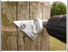
Attach the Mounting Clamp to the pole at the correct position. Care should be taken to ensure that the cable does not infringe the minimum ground clearance requirements under worst case conditions.
