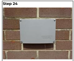
At the building end fit the CBT External Customer Termination Box in a suitable position. This could be inside or outside the building.
