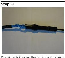
Re-attach the pulling eye to the preconnectorised assembly.
