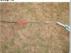
Attach the swivel to the cable using that cable stocking grip.
