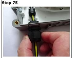
Tighten gland sealing nut.
