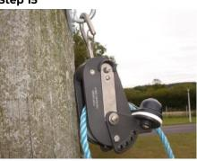
Feed the pulling bond through the pulley at the cable dispenser pole.
