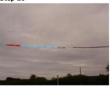
Pull the pulling bond and cable across the span. Care should be taken to ensure that there is no risk to third parties during this operation.
