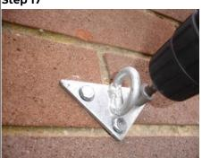
Attach the Mounting Clamp to the house at the correct position. Care should be taken to ensure that the cable does not infringe the minimum ground clearance requirements under worst case conditions.
