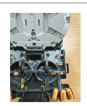
Route the pigtail through the fibre channel up to the required tray. The fibre sheath should be stripped at the tray and stored according to local work instruction.
