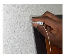
Route Fibre along the external bend manager where necessary.
