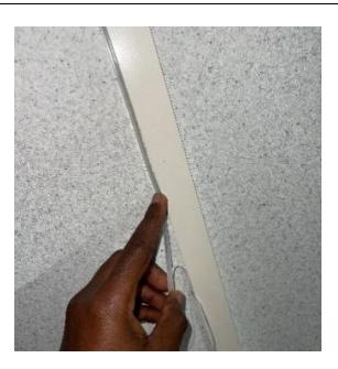
Firmly push the RACEWAY on the surface to hold with place.
