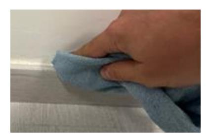
Before installing the RACEWAY on any surface, it is mandatory to clean the surface properly to minimize the presence of dust.
