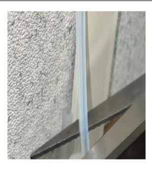
Carefully make a straight cut on the RACEWAY tube when desired length or position is reached.
