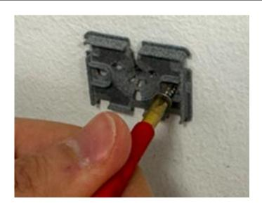
Screw the wall pass-through accessory in on both sides.
