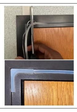
If there is a longer length RACEWAY tube before bend, make a square/perpendicular cut in RACEWAY to flush length with bend manager.
