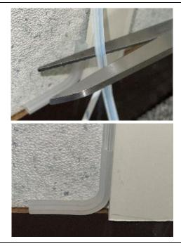
If there is a longer length RACEWAY tube before bend, make a square/perpendicular cut in RACEWAY to flush length with bend manager.
