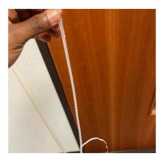
Then take off 20cm of the protective liner to carry on installing RACEWAY.
