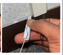
Route Fibre along the flat bend manager where necessary.
