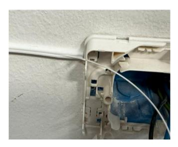
Install RACEWAY and route fibre until wall outlet or wall box.
