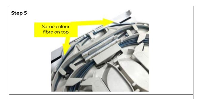
• Ensure that the ribbon fibres enter the tray in the same orientation, this will minimise twists/crossovers in the tray.
