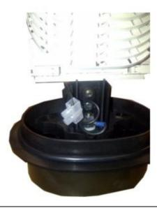
• Store the terminal block into the centre of the joint.
