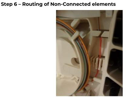
Route the remaining unused elements within the Pull Back Cable around to the right – hand side on top of the tabs, so separating the connected fibres from the non-connected fibres.
