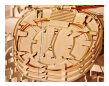
• Manage the spare fibres into the central storage area via the outside fibre track.
