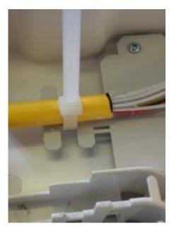
• Refer to section 2 for fitting the split port inserts. Retain cable at both input and output ends with straps cable fixings.
