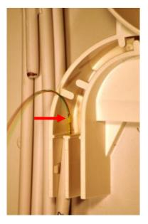
Remove the protective sheath from the BFU to a point 25mm from BFT butt.
