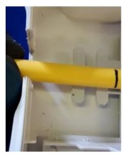
• Place the input side of the COF 201 cable into the bottom port slot and mark the sheath just above the cable retention bracket.
