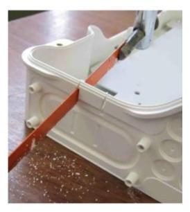
• Saw along moulded guides and snap off remaining material to form a cable access slot at top and bottom of closure left side.
