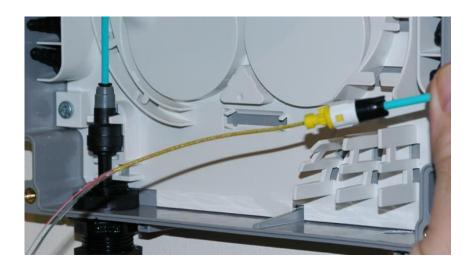
Remove the BFU resin coating to approximately 75mm from the end of the gas block connector.
