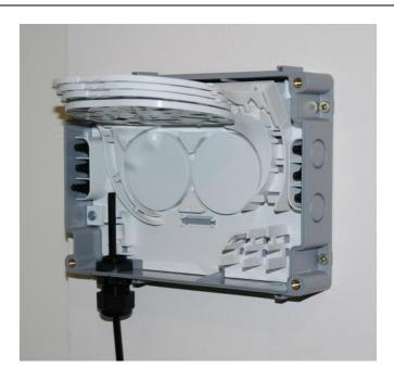
Insert 6mm Blown Fibre Drop (BFD) tube through gland and position approximately 65mm from the lowest face of the box.
