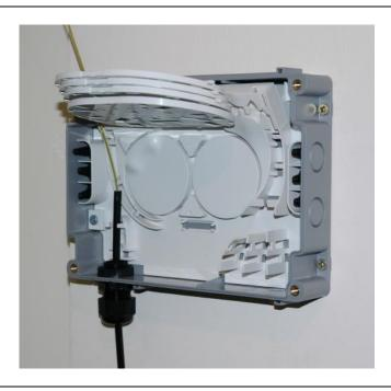
• Install (BFU) using standard BT practices. Ensure a 2m length of BFU is installed beyond the end of the tube.
