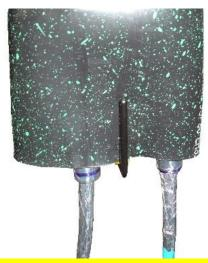
Complete the heat shrinking of the oval sleeve
