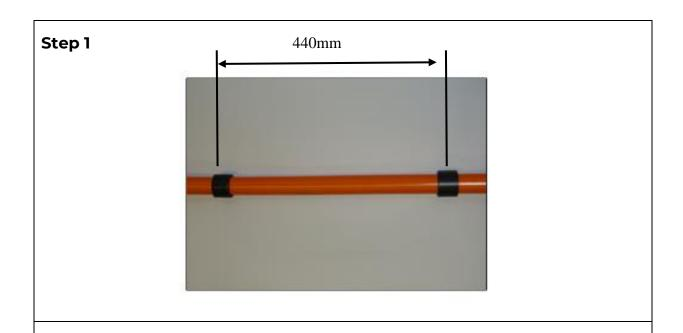
WRAP THE SELF AMALGAMATING SEALING TAPE IN TWO POSITIONS WITH A 440mm SPACE BETWEEN EACH. AFTER ONE COMPLETE WRAP PRESS DOWN AT THE POINT IT OVERLAPS TO SEAL COMPLETELY AROUND THE CABLE. CONTINUE TO WRAP THE TAPE UNTIL YOU HAVE COMPLETED 3 TURNS.
