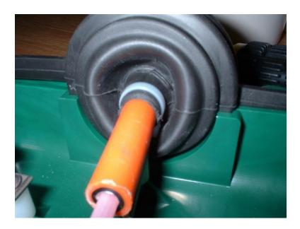
• Push the micro duct back out of the closure so that the end of the sheath sits flush with the end of the clamping plate. Repeat for all other drop ports being used.
