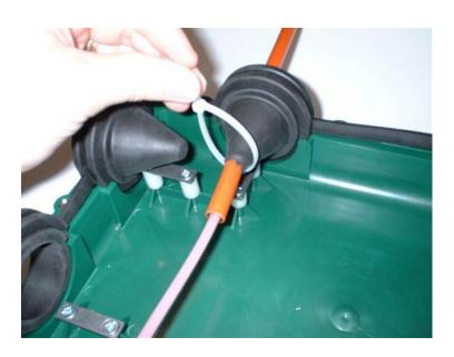
• When using any of the cones; Strip the micro ducts back, leaving enough to make the connection. Feed the micro duct into the closure so that 35mm (1.38") protrudes from the tapered grommet. Secure the micro duct in place by using a cable tie on the grommet as shown.
