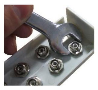
• Fit the uniters to the uniter panel as it is easier to do it at this stage.
