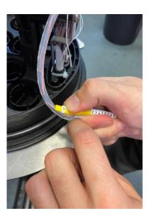
• Add collets onto the spiral wrap to help identify the cable.
