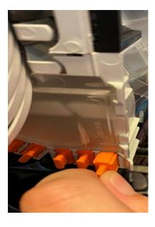
• After preparing the cable for fibre routing remove the retaining block from the closure.
