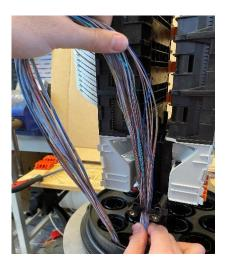
• When installing the ribbon cable into the oval port, make sure to store the fibres into the storage section of the closure.
