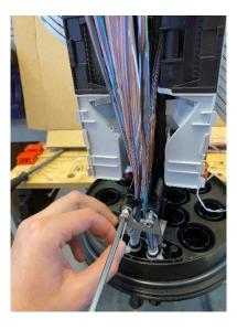
• Place the screws into the metal plate then wrap the binding strings around the screw to ensure the ribbon cable into position.
