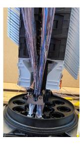
• Bring the oval port seal towards the closure and ensure that the metal plate is aligned with the screw holes.
