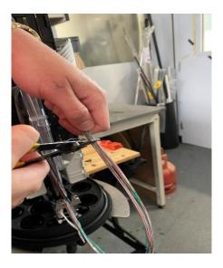
• After you have identified what cable to bring from the loop storage to the splice tray, remove the complete loop of fibre and cut in the middle. Route the live side to the splice trays.
