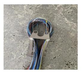
• Feed the loop through metal bracket as shown.
