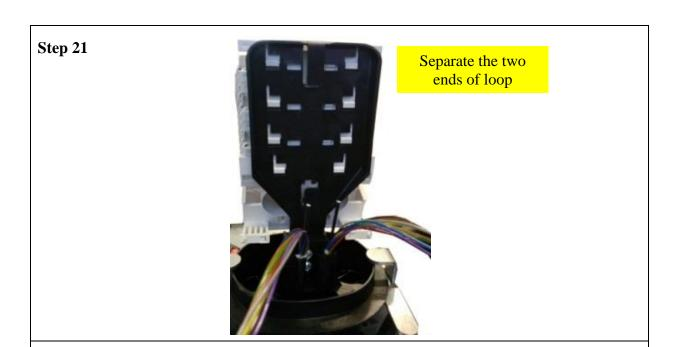
• Firstly, separate the two ends of the loop. Gently straighten the loop away from the CMJ ready to loop into the spine.
