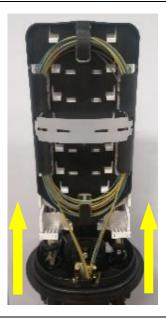
A single loop should be remaining after several coils have been installed.
