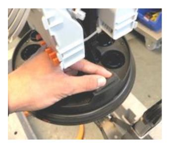
• Push the foam resin stop into the top of the Mobra cavity in the LMJ base, so that it is sat on top of the external MOBRA Bracket inside the LMJ base.
