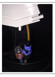
• Fit a tube end cap (BT Item Code - 075146 Blown Fibre Tube 5mm end cap) over the unused tube.
