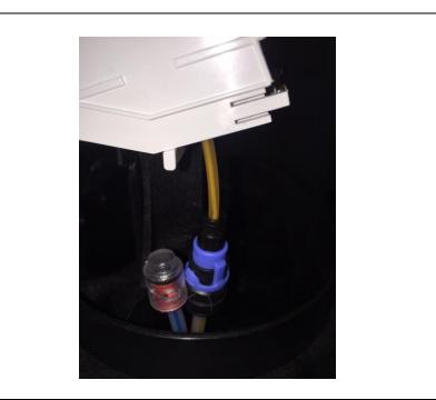
• Fit a tube end cap (BT Item Code - 075146 Blown Fibre Tube 5mm end cap) over the unused tube.
