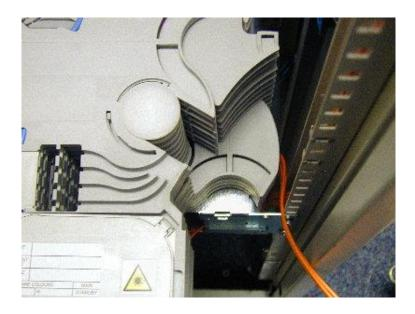
• Identify the required Splice Module (2) and open several of the Splice Modules above it to gain access to the jumper cable feeding area.
