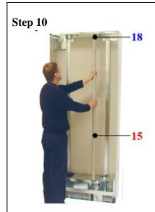
Align the top of the pole with the lefthand side of the left tab in the Top Frame and secure with an M6 screw.
