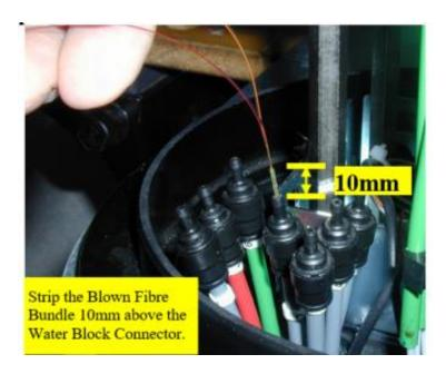
• Strip the Blown Fibre Bundle to expose the fibres 10mm above the top of the Water Block Connector.
