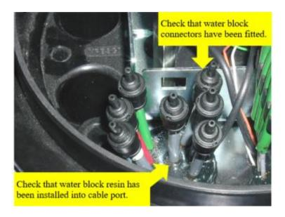
• Ensure that the cable has been installed correctly and that Water Block Connectors have been fitted to all the Blown Fibre Tubes.
