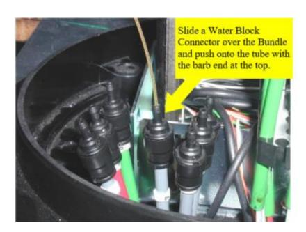
• Slide <u>a new</u> Water Block Connector over the Bundle with the barb end uppermost and plug it onto the Blown Fibre Tube.
