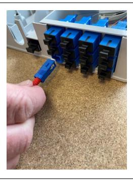
• Before removing anything Begin removing the black plug, then by using the approved fibre cleaning kit, clean both the tail and the port connector.
