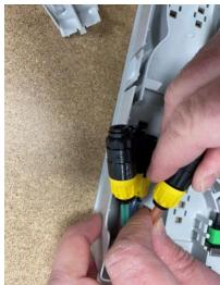
• Feed the cable into the funnel from the outside in and feed the blown fibre tubes into the 5mm gas block connector.
