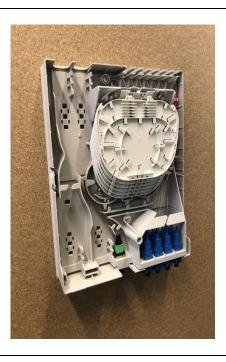
• Now fully tighten all the screws, ensuring the UFS is level and positioned correctly.
