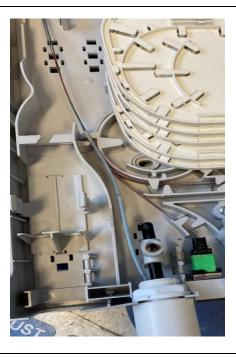
• Slide the cable previously prepared into the funnel and clamp the central strength member down.
