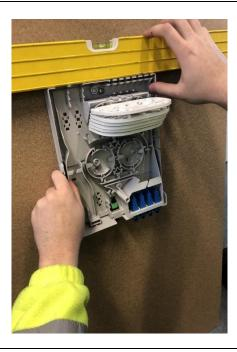
• Ensure that the UFS is level using a spirit level before continuing.
