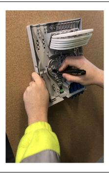
• Then begin marking out the other holes using a marker.
