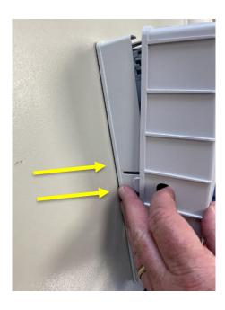
• Begin the wall mounting installation by removing the cover from the UFS, gently push the tabs inwards and slide the cover off.
