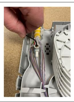
• Use an Allen key to tighten the central strength member clamp.
