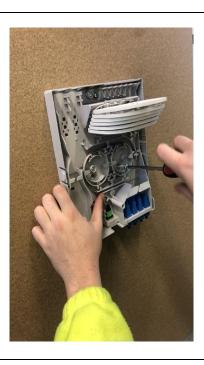
• Insert the screws in the drilled holes, then tighten the screws to 70% tightness.
