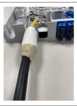
• Insert compound 16 around the funnel and onto the cable.
