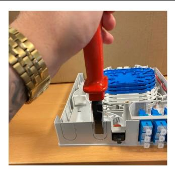
• Begin by removing the lower universal breakout insert using plyers.
