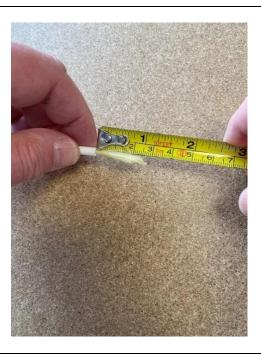
• Begin the process by stripping the cable then by stripping back the aramid to 25mm. The fibre itself is needed to be stripped to a length of 2m from the cable butt.
