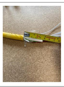
• Mark the cable 1.5m from the end and remove the sheath. Remove all bindings and tape at the butt. Mark the central strength member 45mm from the butt and cut.
