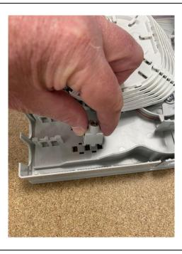
• After removing the breakout slot, you then need to insert the central strength member clamp, align the slots with the slots on the UFS insert and push them into the holes.
