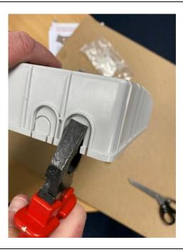
• Begin by removing the breakout, using plyers, apply light force and pull away.
