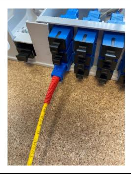
• After the correct measures have been taken, then insert the tail into the patch panel.
