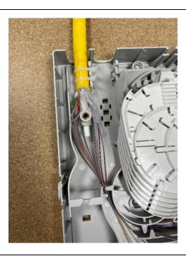
• Insert the cable into the Upper universal breakout. Use cable ties around the butt of the cable to ensure it is in place, then insert the central strength member into the central strength member clamp.
