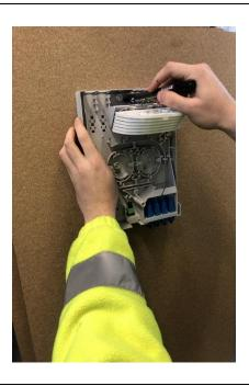
• To start mounting the UFS you need to position it against the wall and mark where a hole needs to be drilled.
