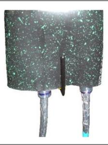
• Fit the glue clip from the Heat Shrink Kit (2) onto the Heat Shrink sleeve between the two cables as shown.
