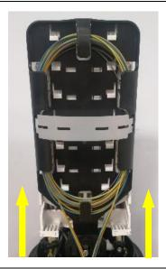
A single loop should be remaining after several coils have been installed.
