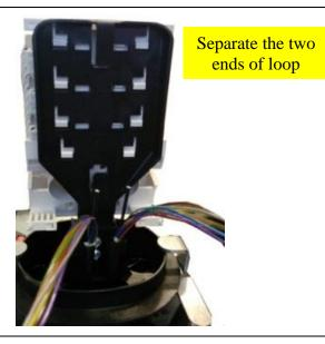
• Firstly, separate the two ends of the loop. Gently straighten the loop away from the CMJ ready to loop into the spine.
