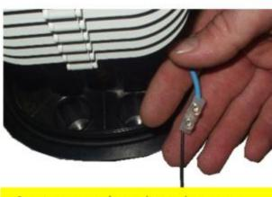
Insert copper conductors into toning connector
