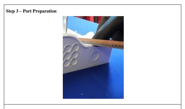
• Saw along moulded guides of the cable ports located at the top and bottom of the splitter DP.
