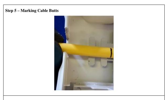
• Place the input side of the cable into the bottom port slot and mark the sheath just above the cable retention bracket.
