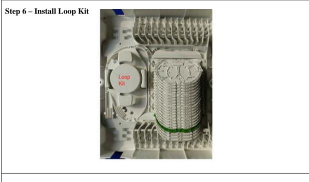
• Install the Loop Kit item code 063238 using the two mounting screws provided.
