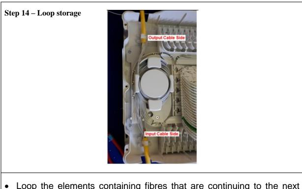
• Loop the elements containing fibres that are continuing to the next floor level into the loop storage area.
