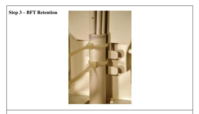
• Retain to the retention lugs in the base of the closure using the large cable ties supplied.
